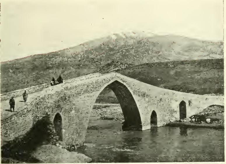
Old Bridge over the Jihon on road to Zeitun.
